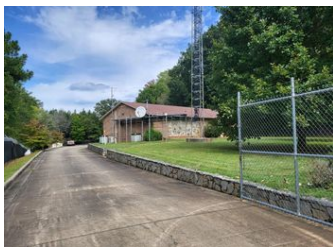
Current Backup EOC
