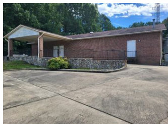
Current Backup EOC
